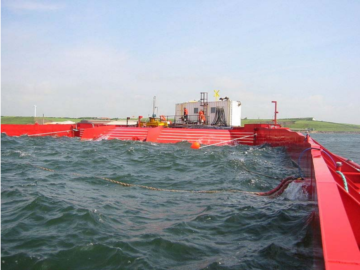
Wave Dragon seen from reflector, prototype 1:4½
